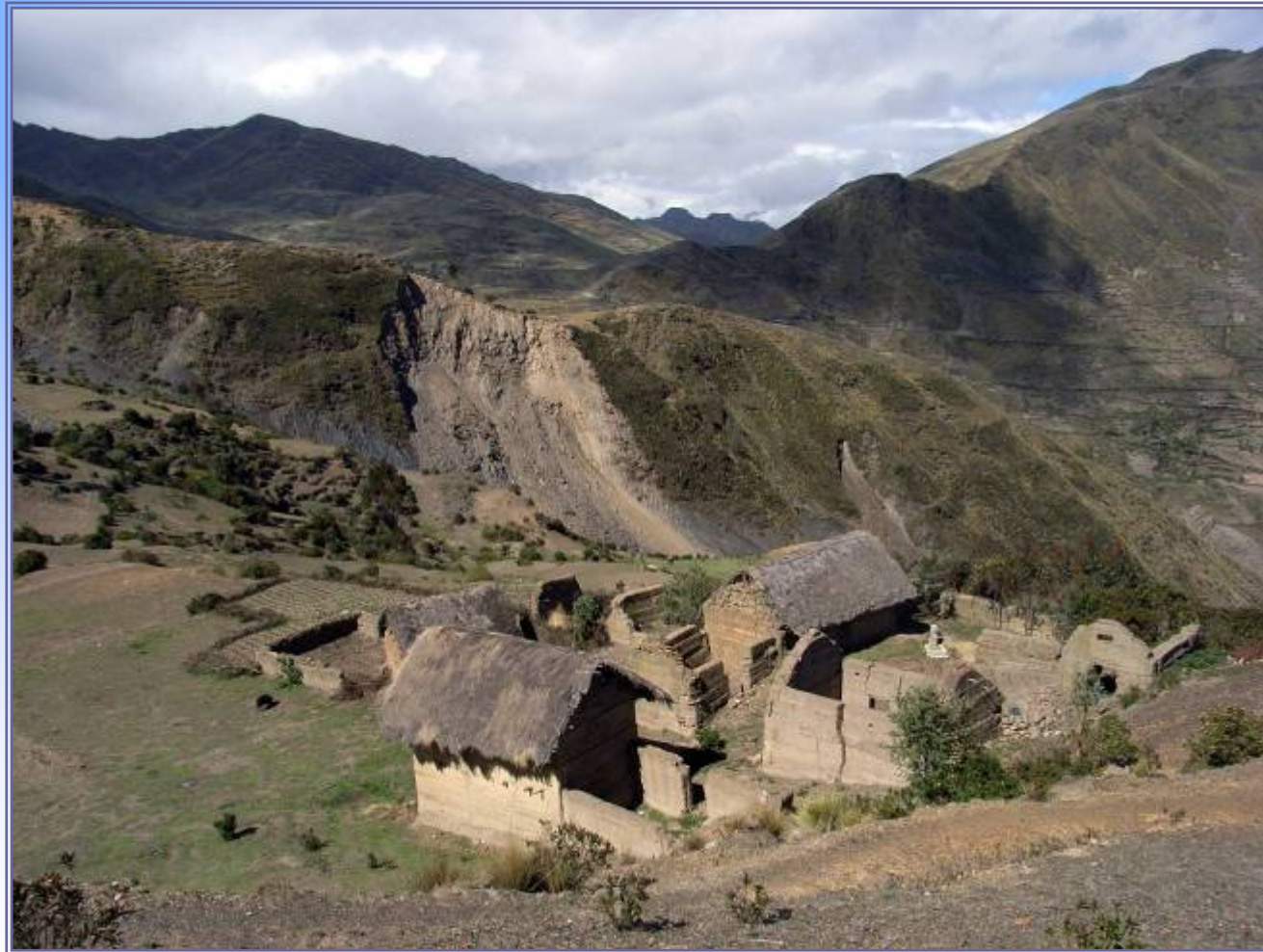
Landslide threatening Totorani Community, Ayata Municipality, 2006.
